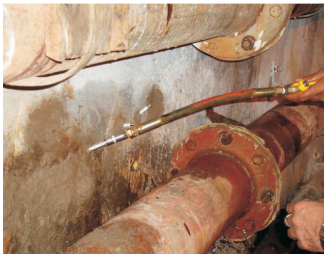
Figure 12: Process of polymer impregnation.
