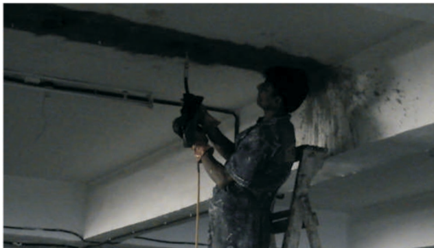
Figure 7: Epoxy Injection in progress.
